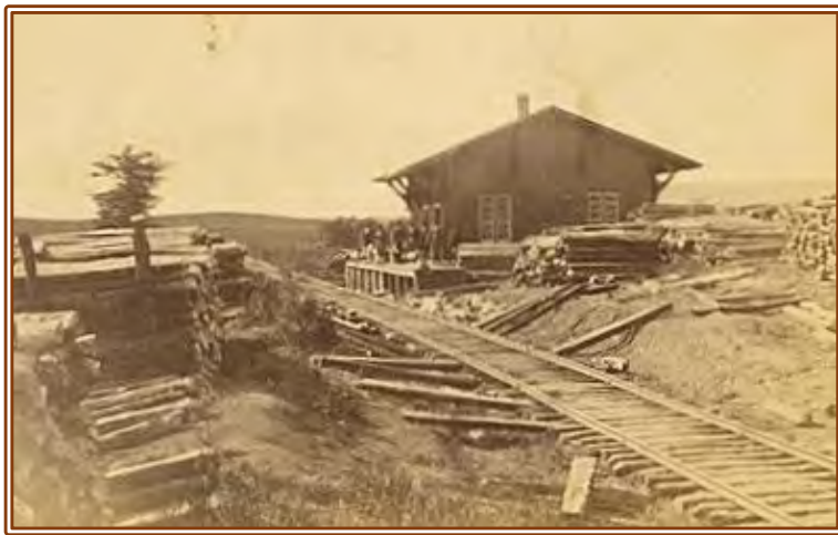
Union Pacific Depot in Tonganoxie under construction
