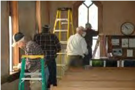
Once the sashes were cleaned, it became evident that some repairs were needed. John Wood took sashes back to his workshop to replace or repair sections of rotted wood and brought the windows back for the second day. On the second day, glass was replaced in the sashes. Much of the existing glass in the windows went right back in the sashes, but replacement glass was also needed.
