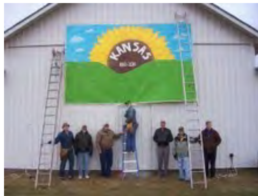
Wednesday workers install new banner on north wall of barn. L-R: Del Englen, Delbert Felts, Dan Carr, Larry Ross, Howard Fields, Lloyd Pearson, Ed Slawson.
